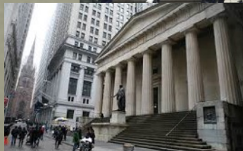
The Custom House, Wall Street, NYC, Ithiel Town, 1837-1842
