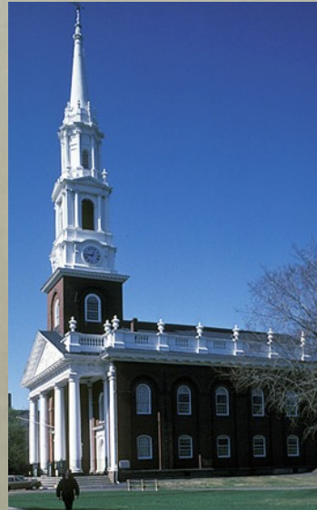
Center Church, Ithiel Town, 1810-1814, photo c. 2010 (at right also clearly shows balustrade at roofline)
