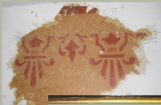
Original wall exposed beneath sheet rock (left) with stencil pattern uncovered.
