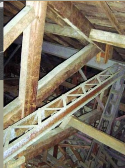
Trinity's attic, steel Inserts, early 20 th c (photo by Joe Dzeda)
