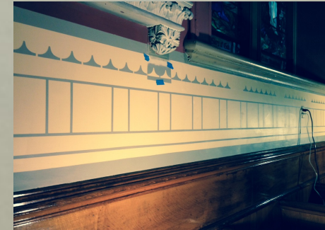
Scallop Stencil Almost Done, Second Bay Ready for Rest of Stenciling, July, 2014
