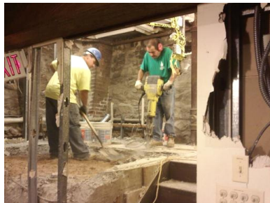
Demolition of the Ladies Room.
